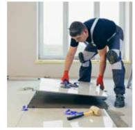
Note: Larger tiles may require a thin layer of adhesive on the back of the tile as well Check it with a spirit level
